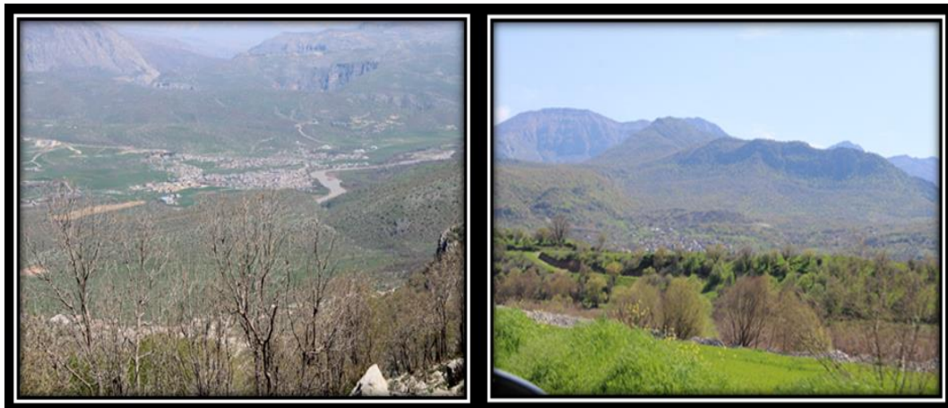
Picture (2-3) Shows some areas of immersion inside the reservoir Bakhme Dam
