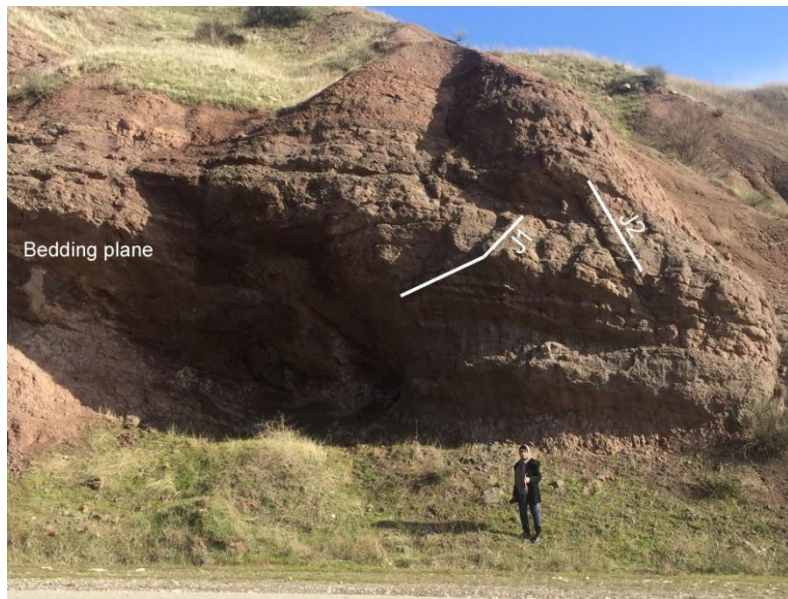
Fig. 6: General view for slope at station no.1 with marked discontinuity sets
