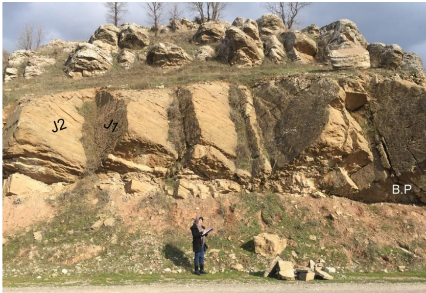
Fig. 10: General view for slope at station no.3 with marked discontinuity sets
