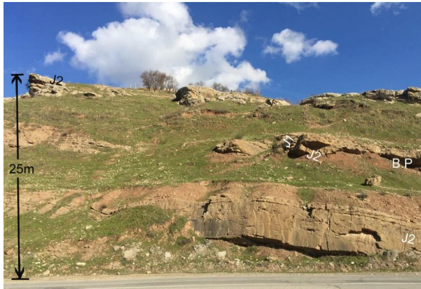
Fig. 8: General view for slope at station no.2 with marked discontinuity sets
