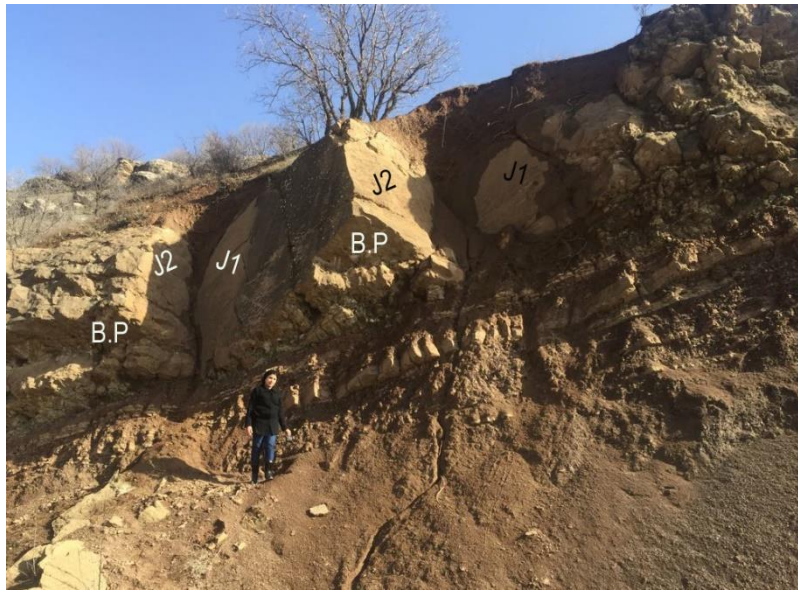
Fig. 16: General view for slope at station no.6 with marked discontinuity sets
